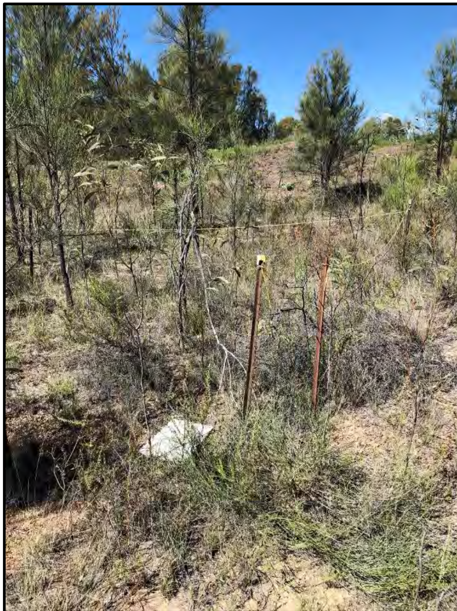
An example of dilapidated barricading at HVO-76
