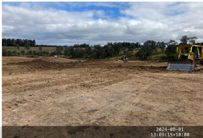
Contour construction at East TSF Rehabilitation Area
