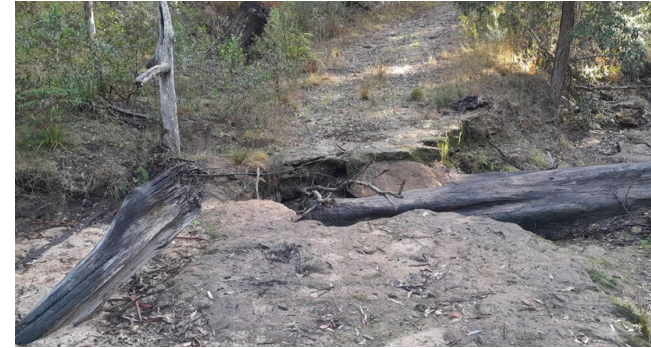
Erosion repair – Condon View
