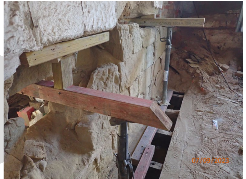
Temporary structural support at Archerfield Homestead distillery
